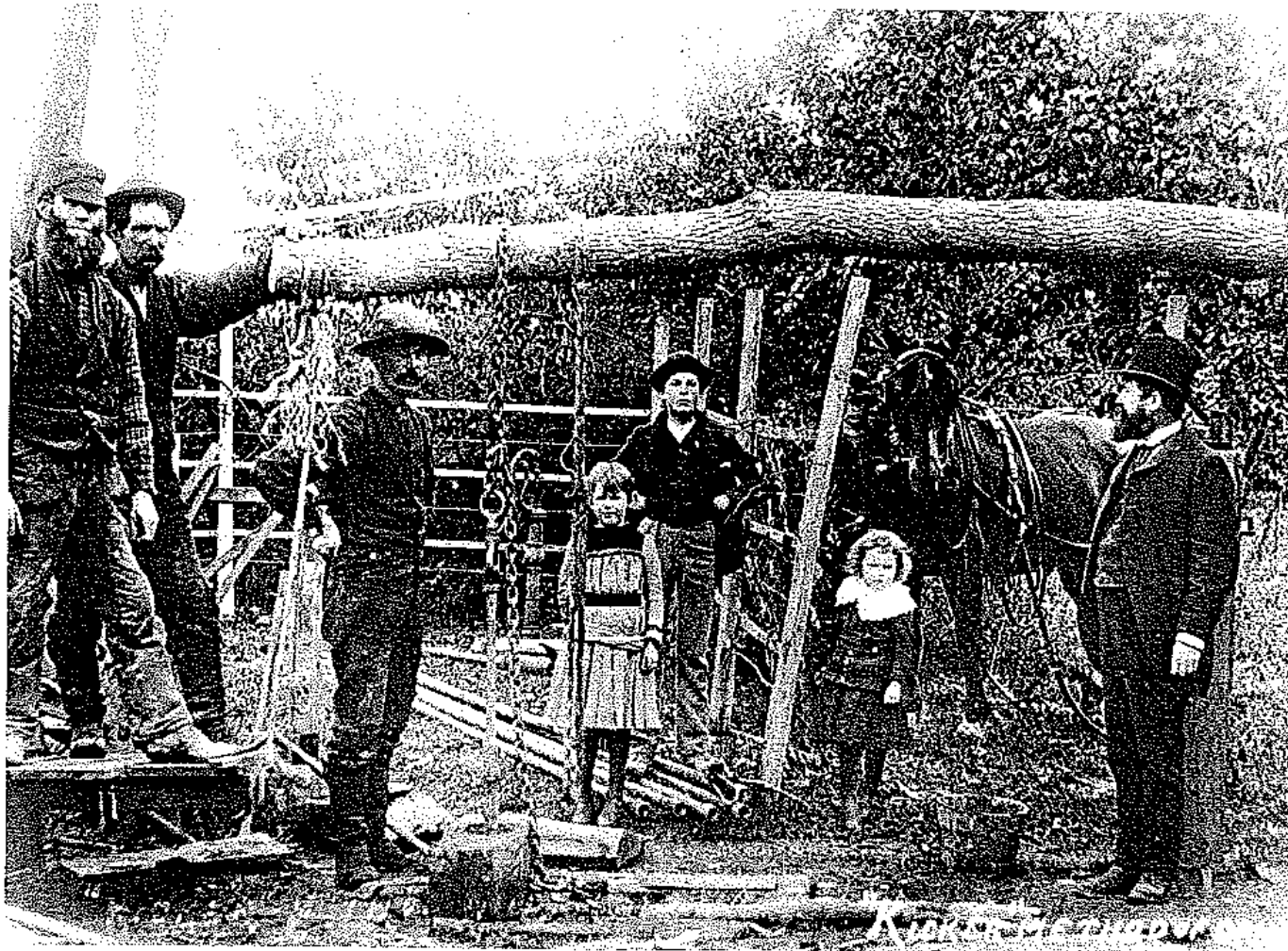
Williams probably used this "kicking or spring pole method" for drilling his wells
